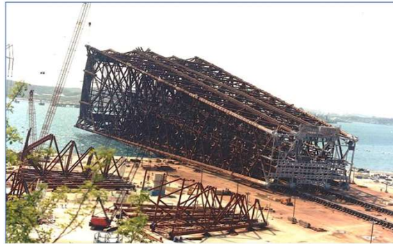
Figure 1(a) Schematic of a generalized offshore oil and gas platform. Adapted from Manago and Williamson (1998). (b) Construction of jacket support for oil platform offshore California. Note size of crane and large trucks compared to the size and configuration of underwater support for offshore platform
